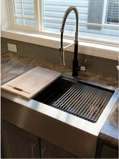
UK3 Sink & Faucet
